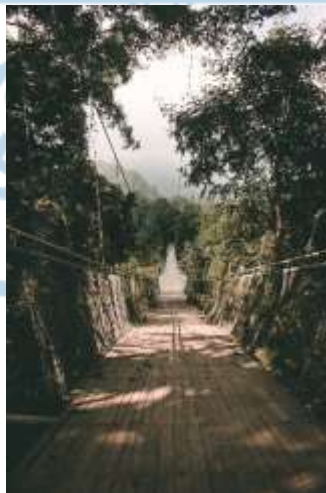
Gambar 1.1 Foto Situ Gunung Suspension Bridge
