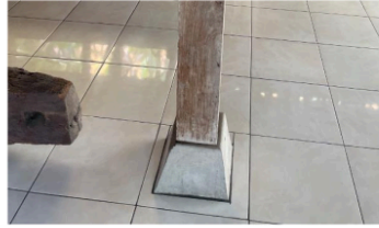
Figure 5. Timber column to the base of the existing building
