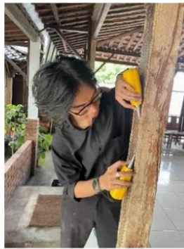
Figure 8. Non-destructive test on one of the side columns using the indirect method
