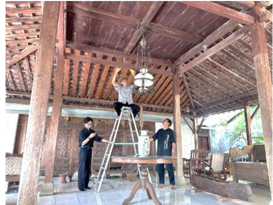
Figure 6. Non-destructive testing to obtain the MoE_{dyn} of Joglo existing building
