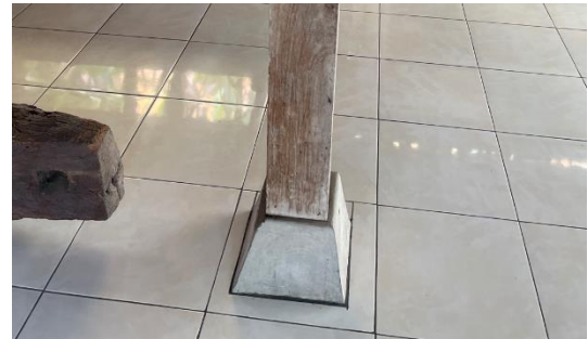
Figure 5. Timber column to the base of the existing building
