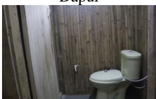
Gambar 14. Tahapan Finishing Kamar Mandi
