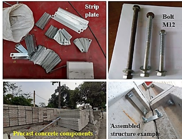
Fig. 2: Examples of some structural components photographs.
