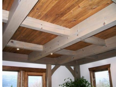
Figure 2. Timber floor slabs [9].
