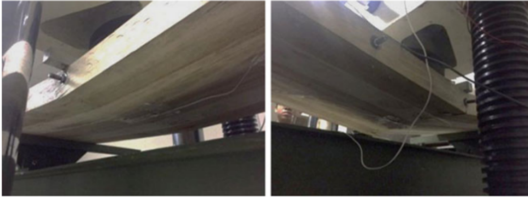
(a) Simple tension failure of S20-B01. (b) Simple tension failure of S20-B02.
