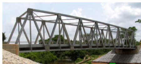
Figure 1 Truss Steel bridge [5].
