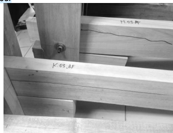
(a). Meranti timber connection.
