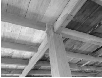
Figure 2. Beam-column joint connection of Minahasa Traditional House: Interior joint.
