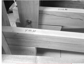
(a). Meranti timber connection.
