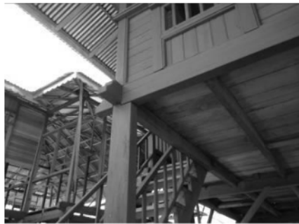
1 Figure 1. Beam-column joint connection of Minahasa traditional house: Exterior joint.
