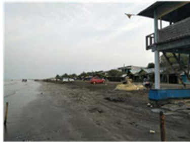
Figure 2. Coast guard structure at Samudra Baru Beach
