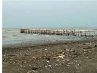
Figure 3. Drainpipe at Samudra Baru Beach
