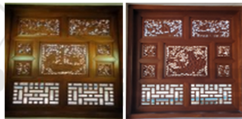
Figure 12: Ventilation openings with hand crafted wooden trellis, decorated with The Three Kingdoms episodes.
