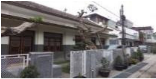
Figure 3: Façade (Basalamah 4, 6, 8) as seen to the east, junction with Jalan Kasmin.
