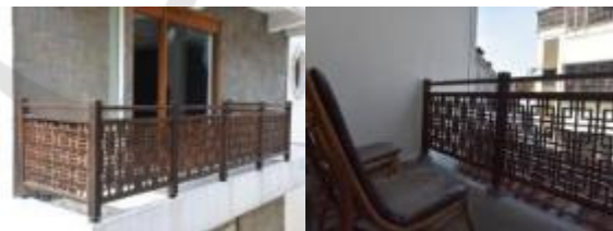
Figure 13: Railings with traditional Chinese patterns, the balcony facing the street in front.
