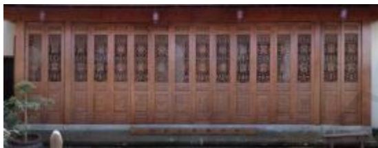
Figure 9: Set of 18 wooden lattice panels at the hall building.
