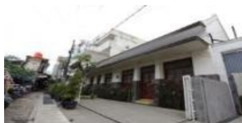
Figure 2: Building (Basalamah 6, 8) façade as seen to the west, the end side of the traditional wet market.
