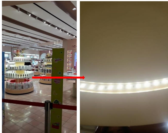
Figure 5. the use of LED lights on the island display in Sociolla Paskal23, Bandung (Sources: Authors Documentation, 2022)
