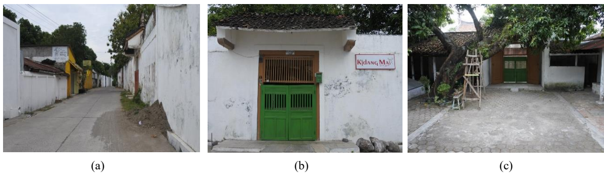
Figure 2. Peranakan House – Kidang Mas, Babagan, Lasem. (a) Surrounding the house; (b) The house gate; (c) Inside the house complex.
