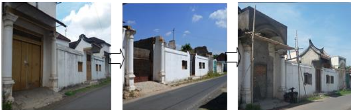
Fig. 13. The Issues in Pecinan, Lasem – Dismantled
