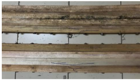
Figure 4. Failure type of the beam for all beams specimens which are simple tension.
