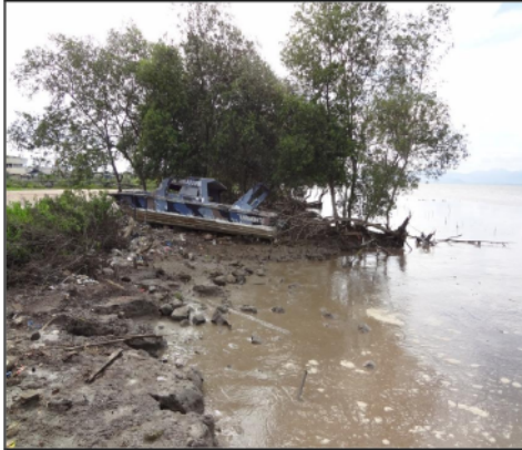
Figure 10 Conditions Shorelines eroded at Karangantu's coastal area
