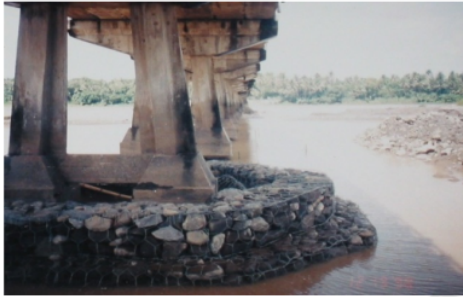
Figure 2: Example of riprap around the pier (From: istiarto.staff.ugm.ac.id).
