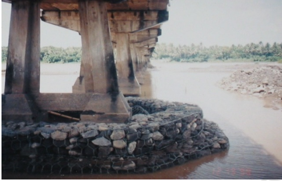
Figure 2: Example of riprap around the pier (From: istiarito.staff.ugm.ac.id ).
