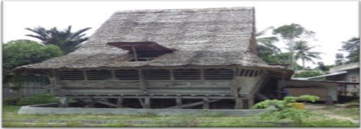
Figure 1: Front side of traditional house in Bawolato. Source: Researcher document
