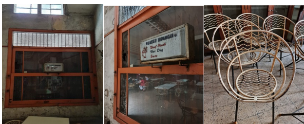
Picture 31-33. Sliding window in the restaurant area with stained glass and signage. Right picture shown restaurant chairs in good shape due to good quality steelwire (source: personal documentation)
