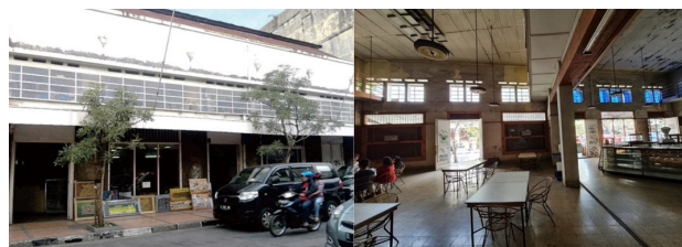
Picture 15-16. The façade of shops no. 22 & 24. Both shops has a slight different style as the bakery on no. 24 has two entrances with big glass window in the middle and the restaurant on no. 22 has two big sliding window with one main entrance in the middle
