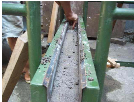
Gambar 4. Proses pengecoran dinding.
