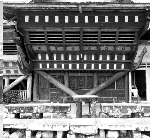
Figure 6: A house with a substructure adjustments
