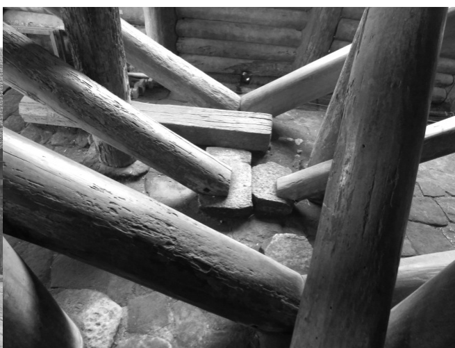
Figure 4: The slanting piles base of the noble house
