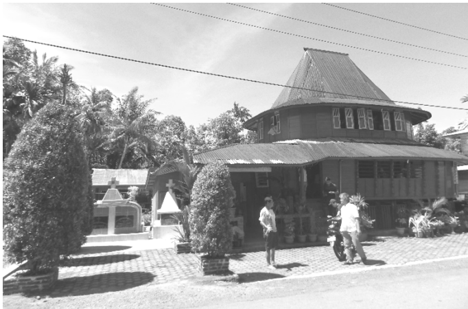
Figure 5: A 2 storey house with roof adjustments
