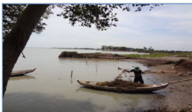
Fig. 7 Erosion at East Lontar's coastline
