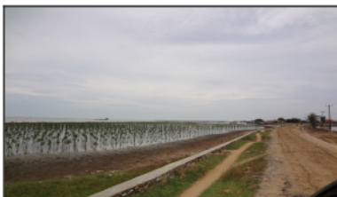
Fig. 9 Condition Lontar's coastline protected by breakwater parallel to the beach combined with early mangrove plant
